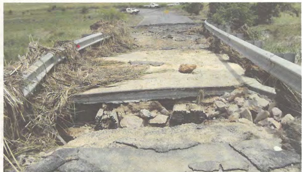
Bridge at Woodville Road
