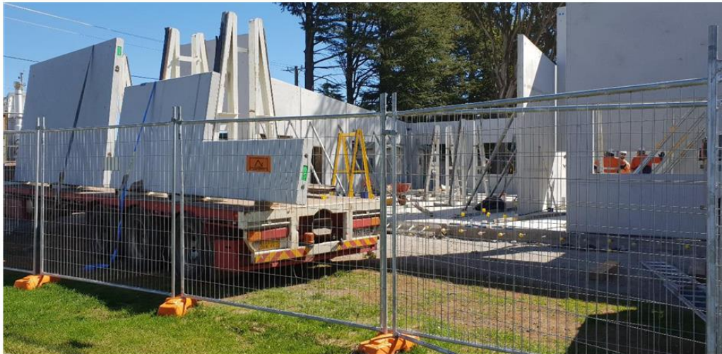
Delivering and installing tilt up panels
