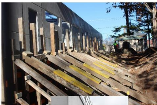
Veranda formwork and concrete
