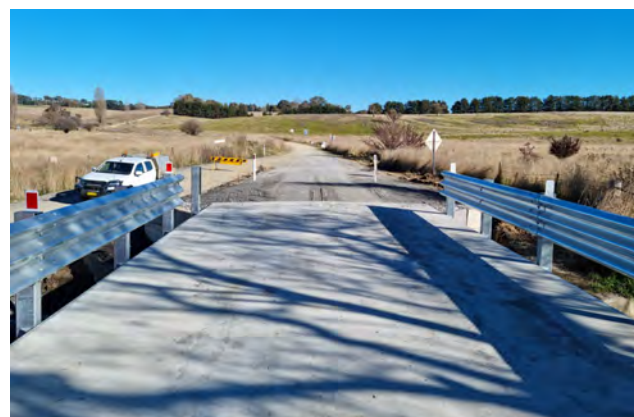
Woodville Road Bridge, Crookwell River
