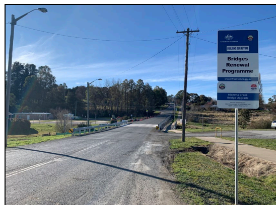
New Kiamma Creek Bridge
