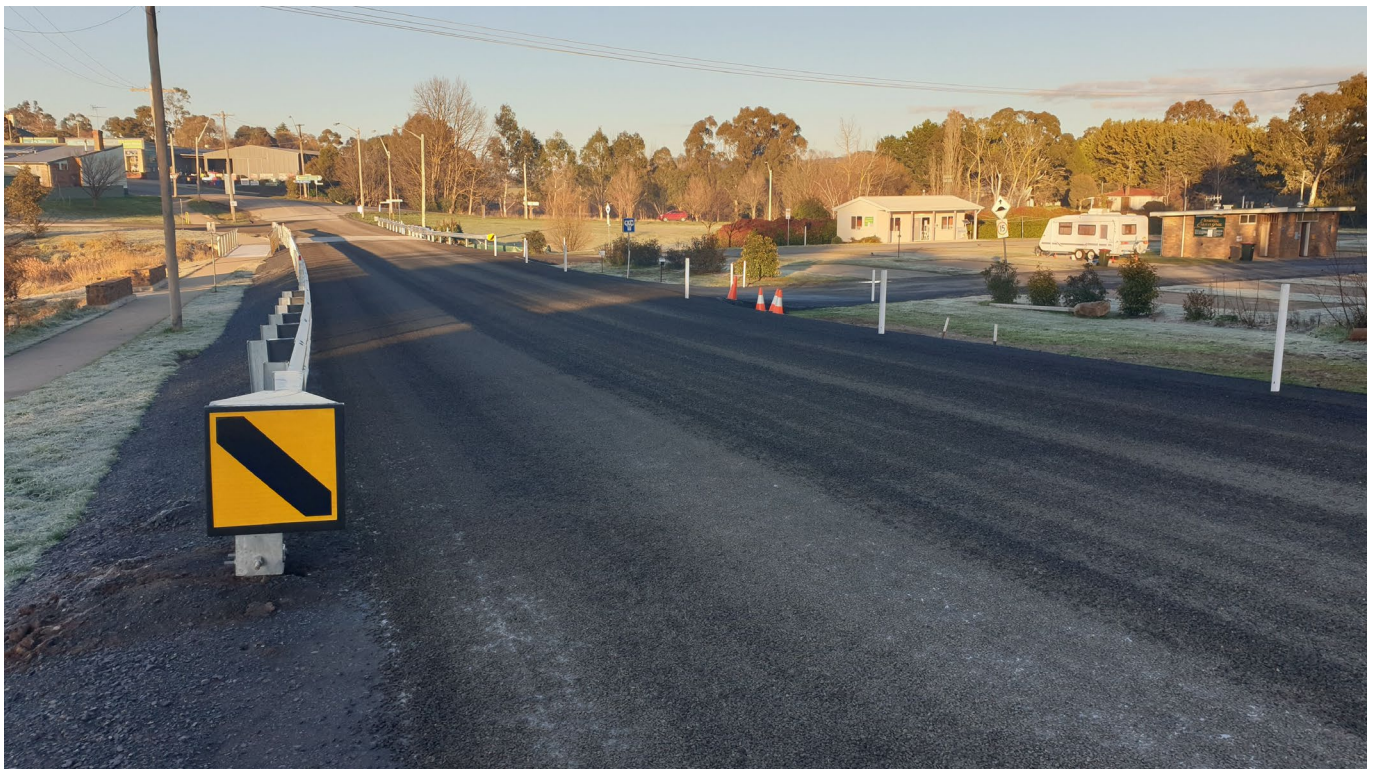
Kiamma Creek Bridge upgrade
