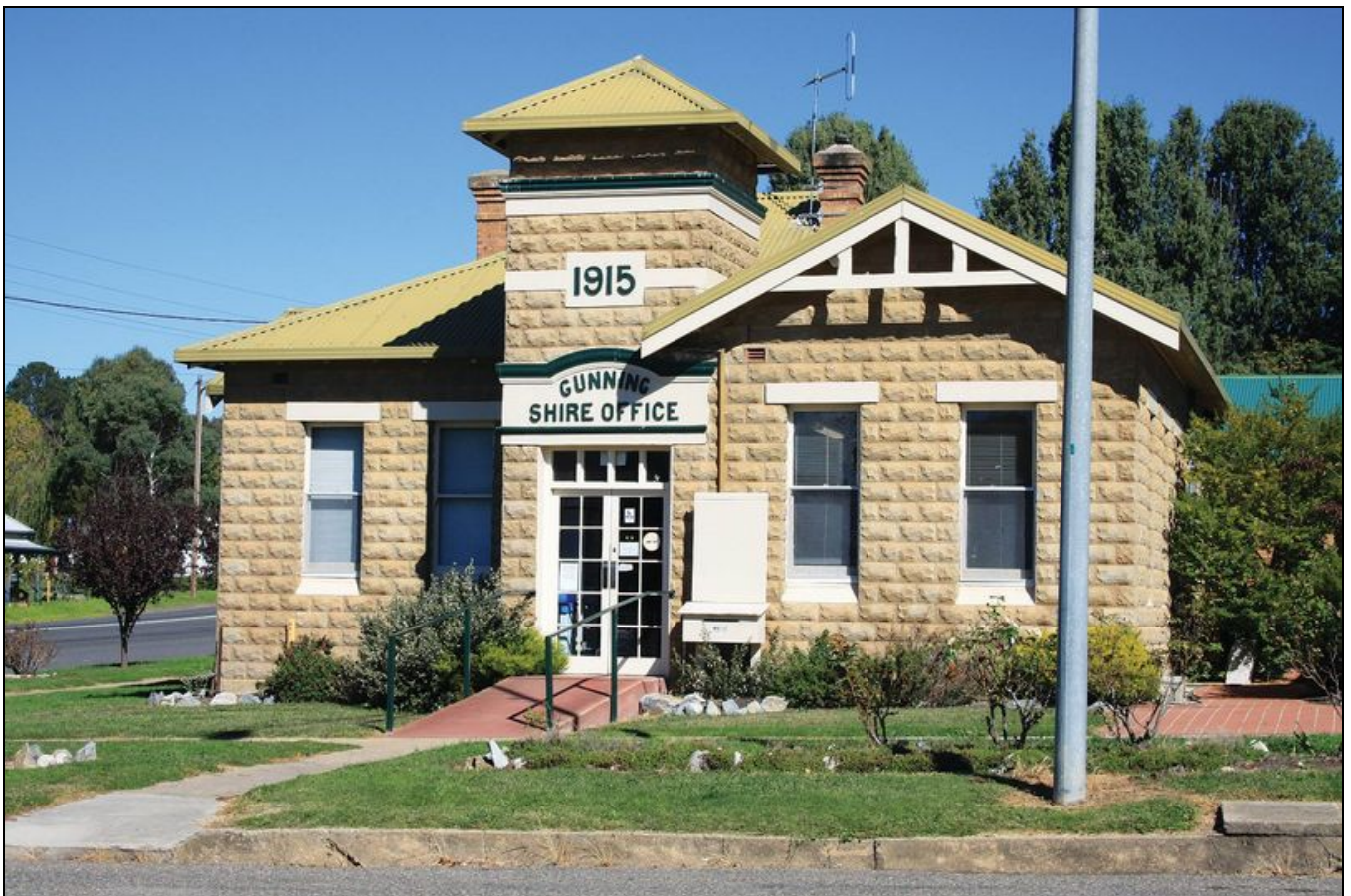
Gunning Administration Office
