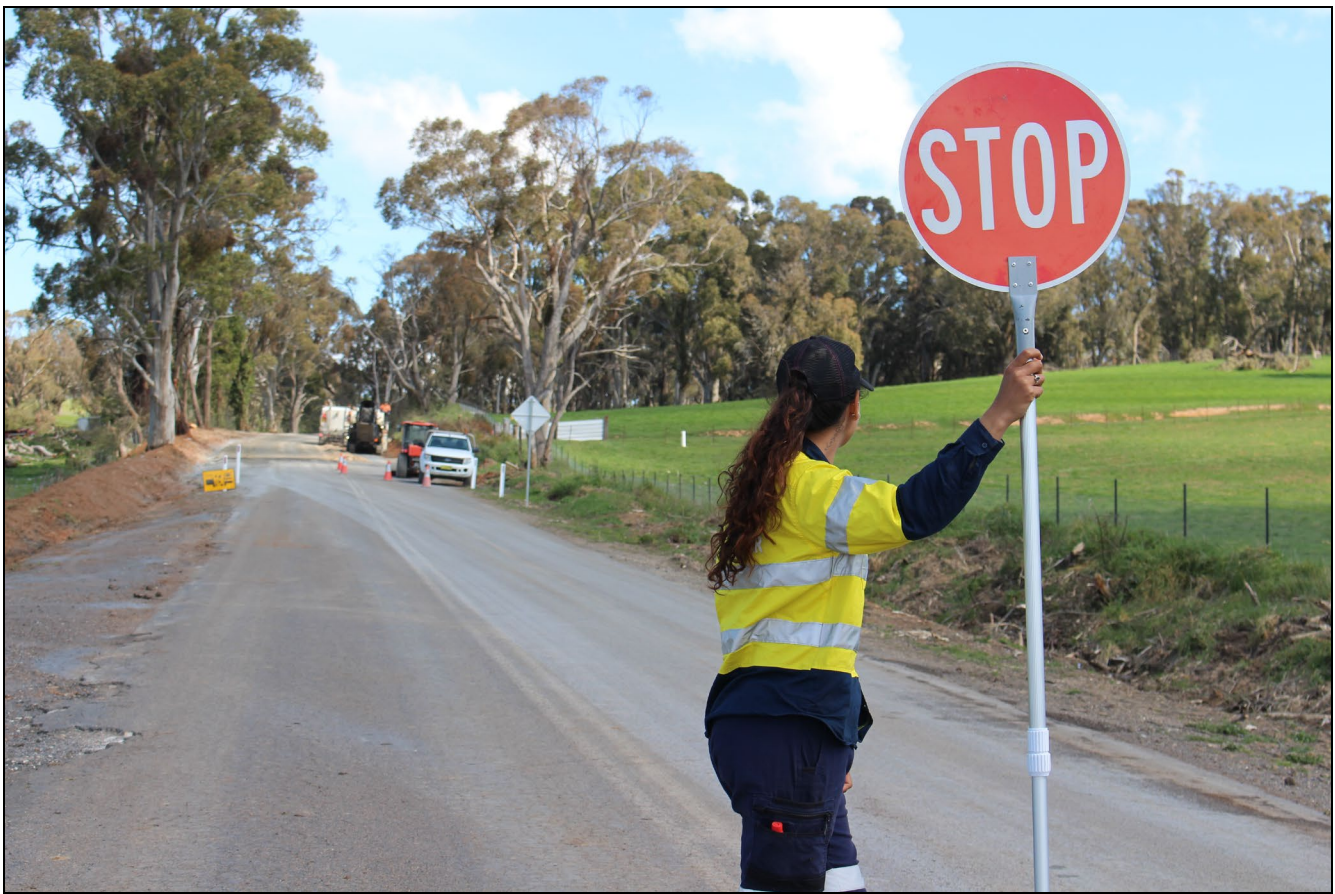
Work on the Grabben Gullen Road MR52
