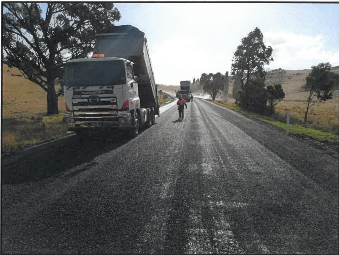
Work on the MR52 Gunning Road Devil's Elbow section road reconstruction
