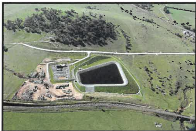
Gunning Water Filtration Plant was completed in 2014
