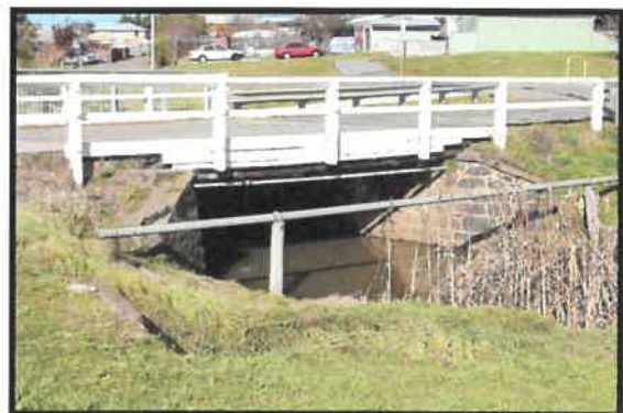
Kiamma Creek Bridge
