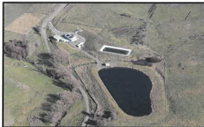
Aerial view of Taralga Sewerage Treatment Plant
