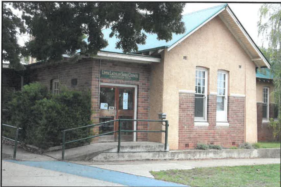
Crookwell Administration Office
