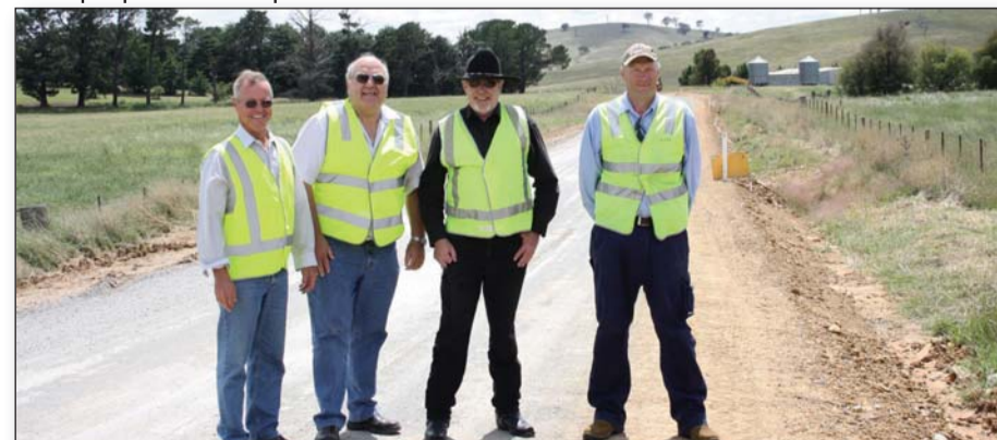
Inspecting the rehabilitation road works in progress by Council staff on Jerrawa Road are: (L to R) Clr Shaw; Director of Works, Phil Newham; Clr Searl; Overseer Maintenance - Gunning, Ted Alchin.
