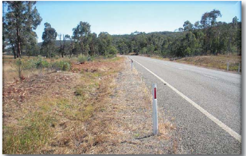
Above: Improved sight distance near Bridge Creek road through to reconstruction works at Junction Point Road.
