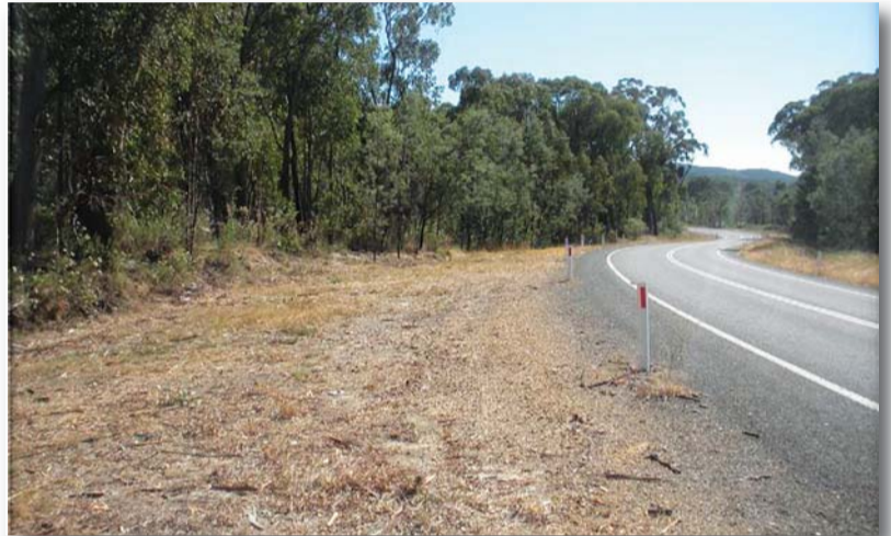
Above: View of the area near Bridge Creek Road where the kangaroos were being hit and killed on a regular basis. The removal of the re-growth, weeds and wattles has improved the sight distance through here allowing the motorist to see any potential fauna hazards.
