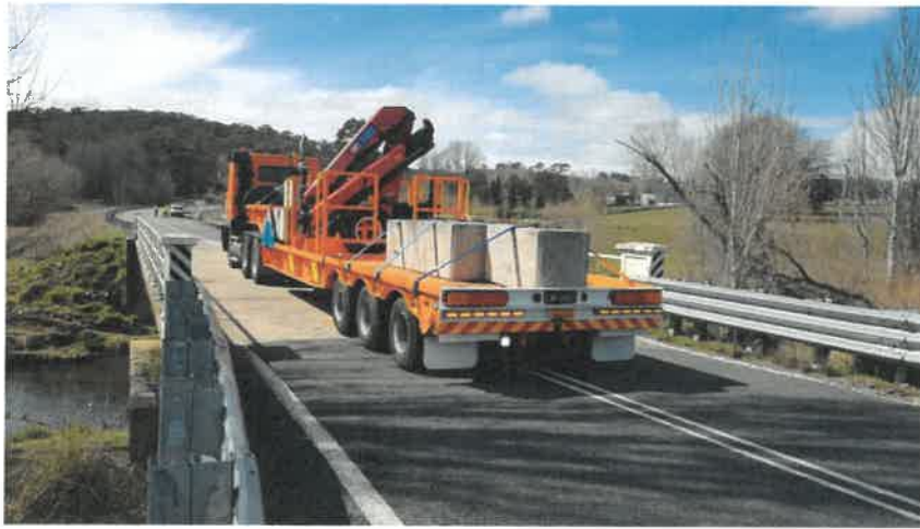
Figure 2- Test Truck at the Bridge Centreline
