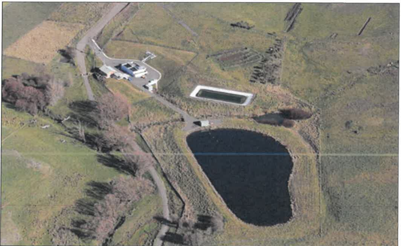
Taralga Sewer Plant
