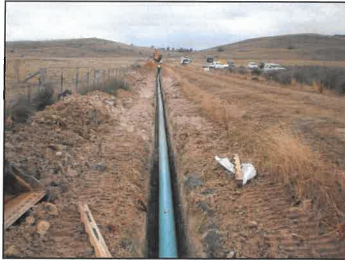
The Gunning-Dalton Water Supply Improvement Project
