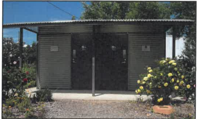
Kiamma Creek Crookwell toilet amenities
