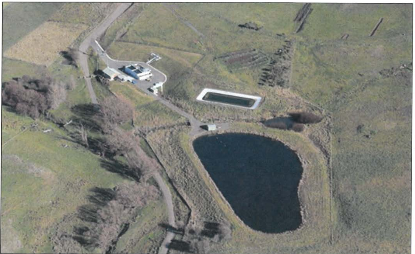
Taralga Sewer Plant
