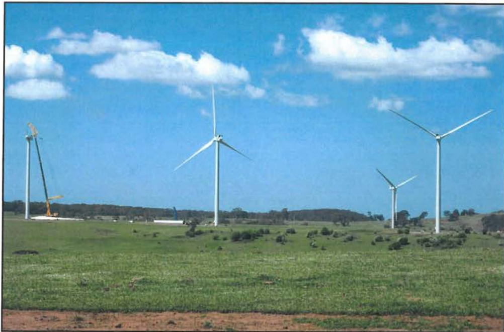
Construction of the Taralga Wind Farm
