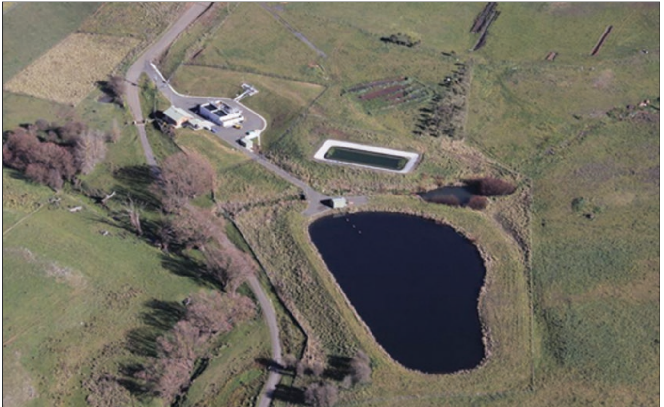
Taralga Sewerage Plant
