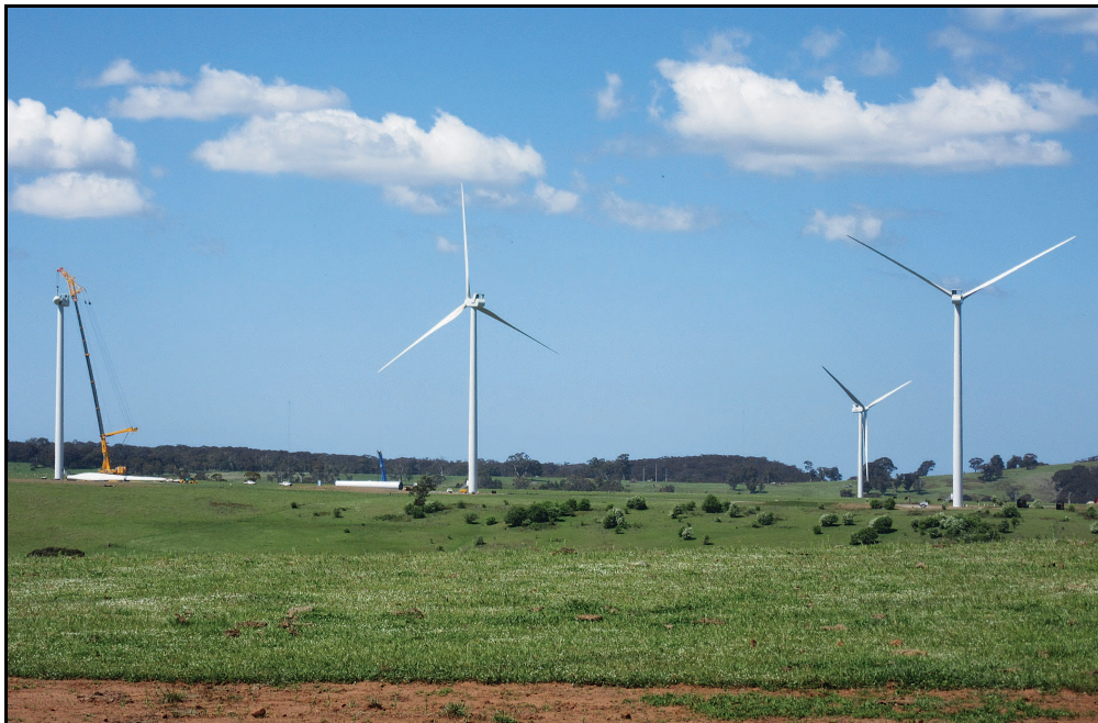
Construction of the Taralga Wind Farm
