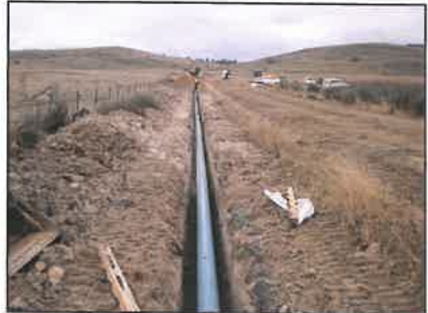
Dalton Pipeline – part of the Gunning-Dalton Water Supply Improvement Project
