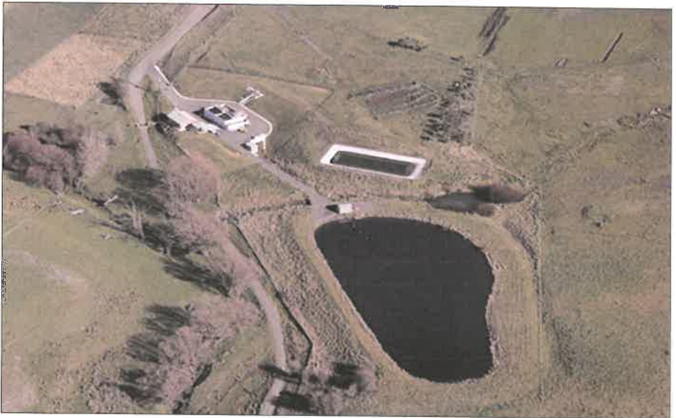
Taralga Sewerage Plant
