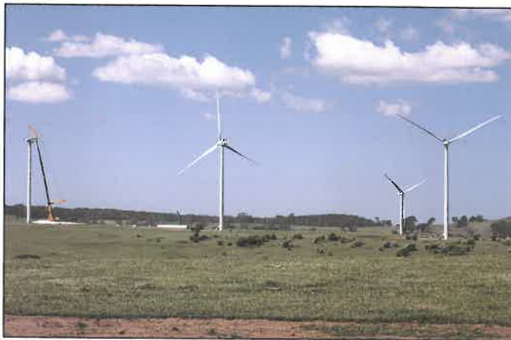
Construction of the Taralga Wind Farm
