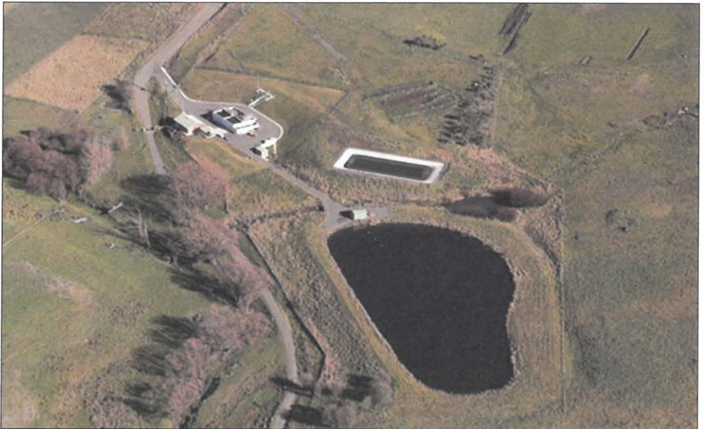
Taralga Sewerage Plant
