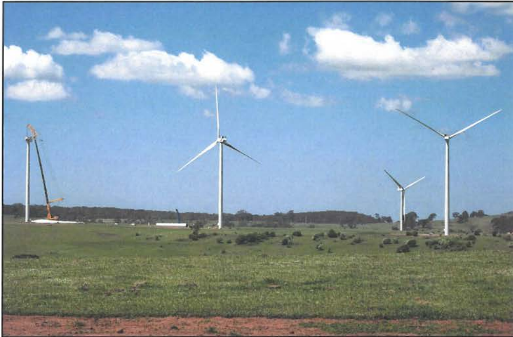
Construction of the Taralga Wind Farm
