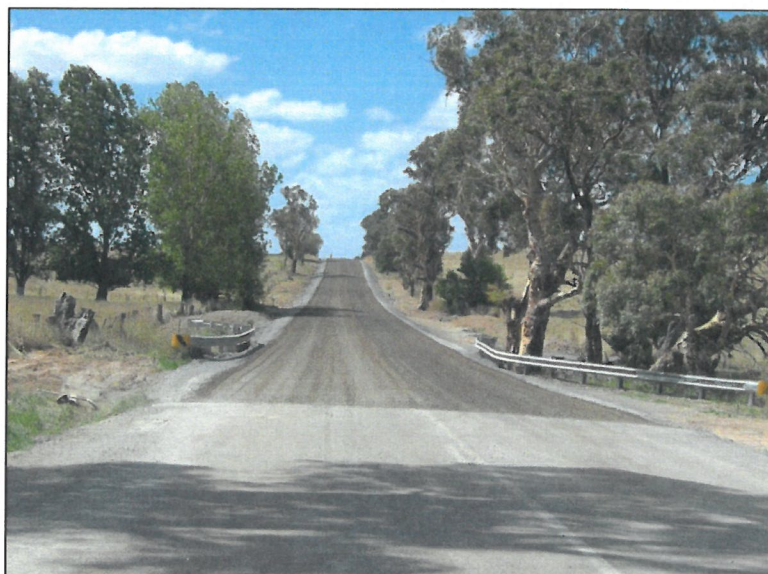
MR52 road reconstruction and bitumen resealing
