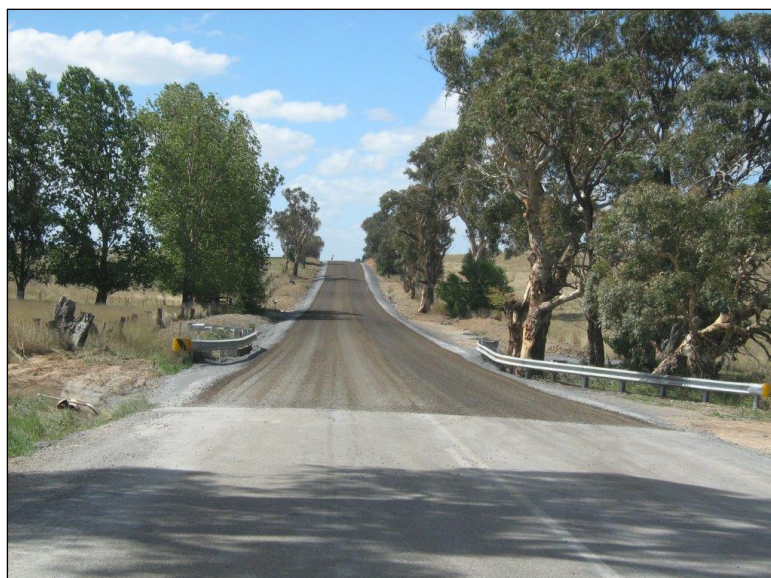
MR52 road reconstruction and bitumen resealing
