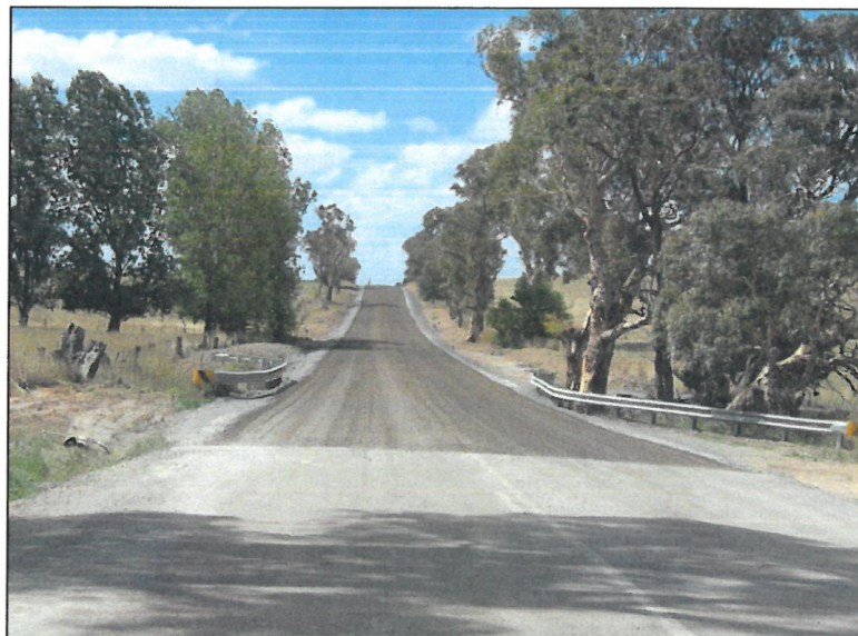
MR52 road reconstruction and bitumen resealing
