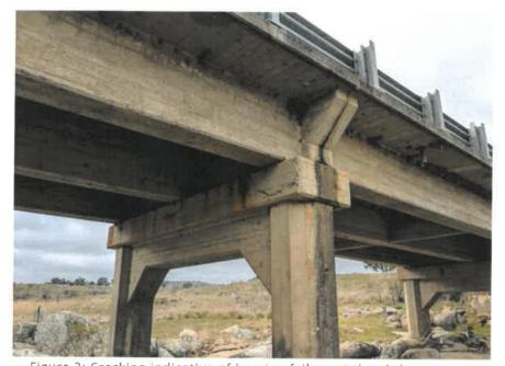
Figure 3: Cracking indicative of bearing failure at the girder support
