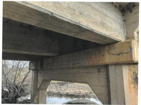
Figure 4: Further cracking indicative of bearing failure at the girder support
