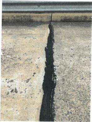
Figure 6: Worn and cracked sealant between bridge spans
