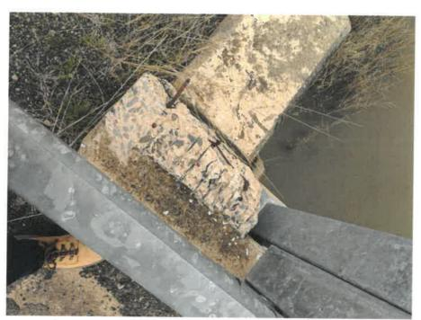
Figure 5: Partial demolition leaving reinforcement exposed
