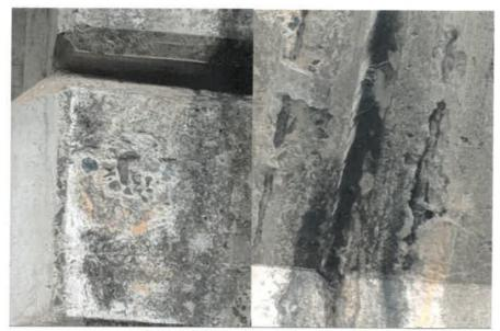
Figure 4: Exposed reinforcement
