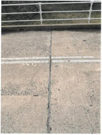
Figure 7: Failed sealant at bridge joint
