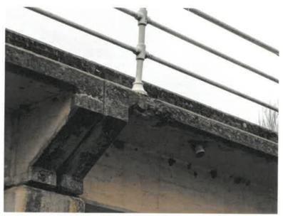
Figure 3: Spalled edge of bridge deck
