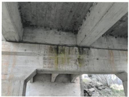
Figure 6: Water intrusion through failed bridge joint seals
