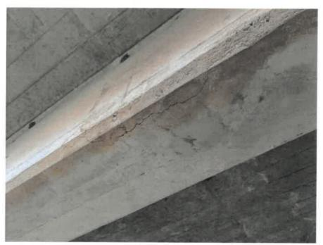
Figure 5: Horizontal cracking indicative of Internal spalling
