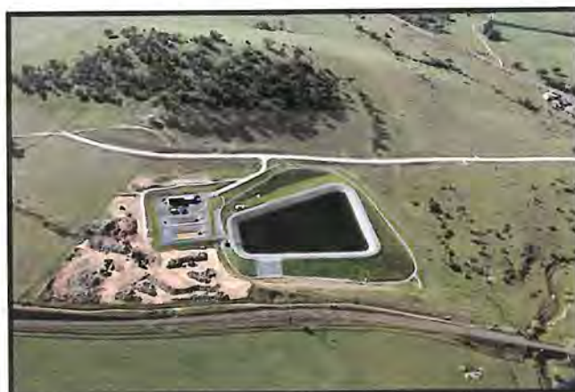
The Gunning Water Filtration Plant was completed in 2014
