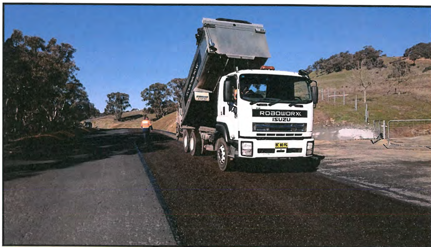
Road resurfacing on RMS State Road MR54
