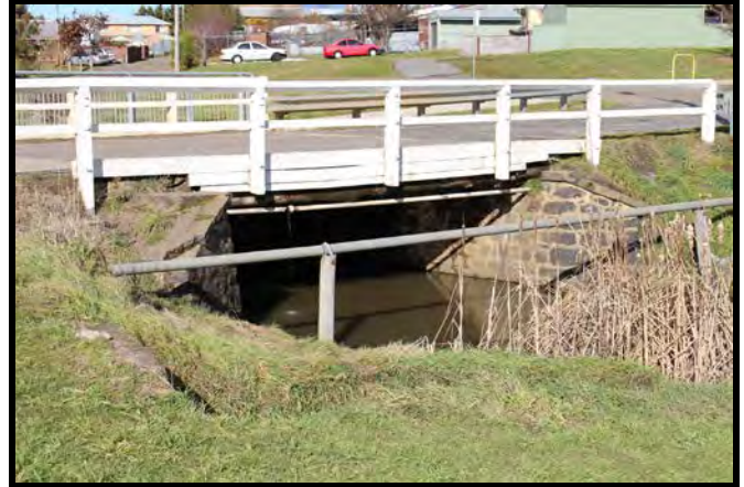
Kiamma Creek Bridge
