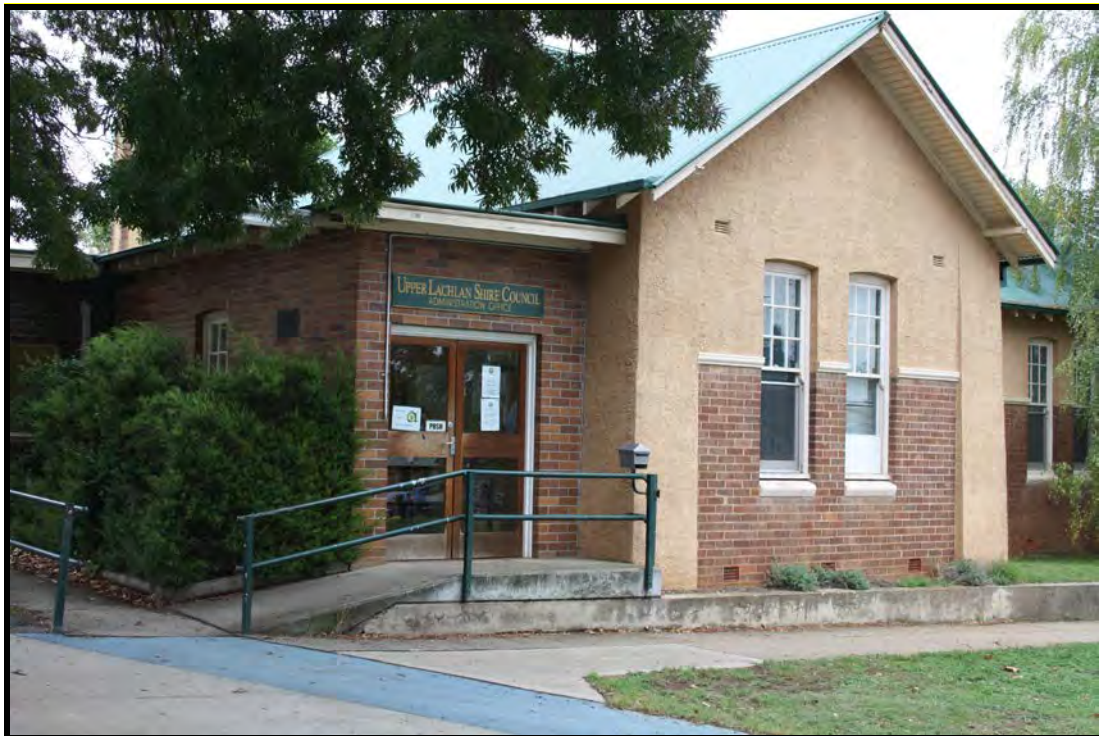
Crookwell Administration Office
