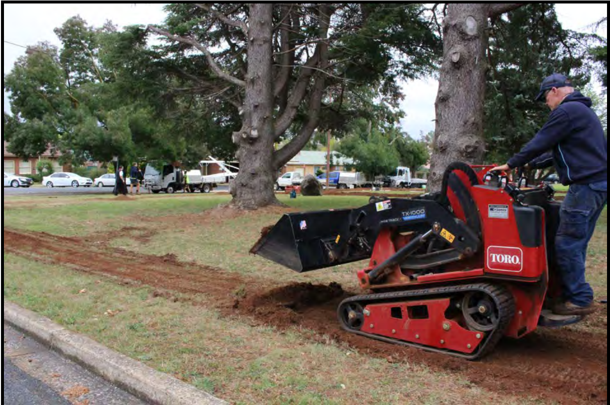
Work on a new irrigation system at Crookwell's Memorial Park
