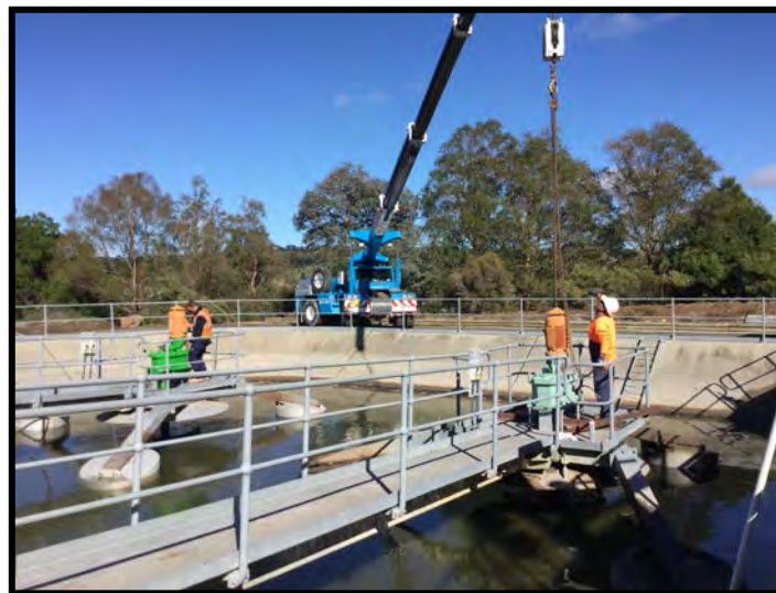
Crookwell Sewerage Plant aerator gearboxes refurbished in April 2017
