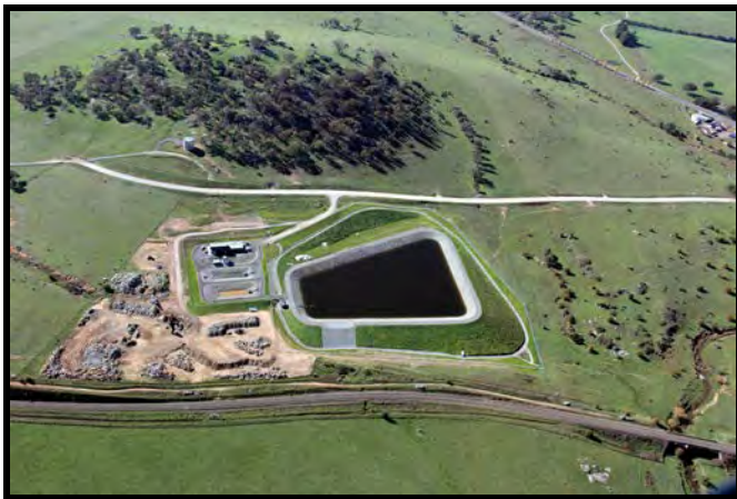
Gunning Water Filtration Plant was completed in 2014
