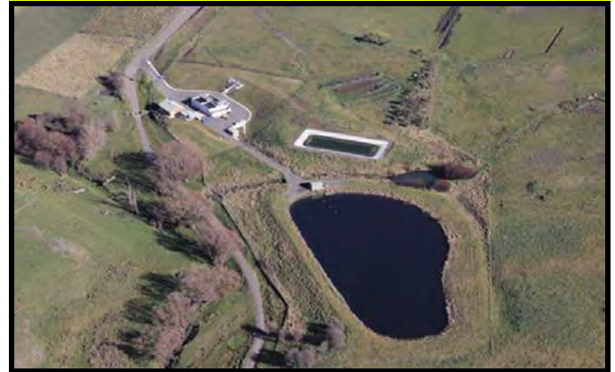
Aerial view of Taralga Sewerage Treatment Plant
